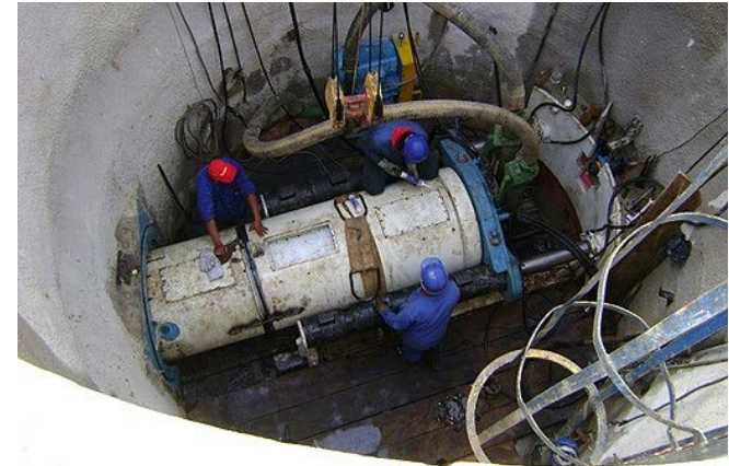
4 to 7 ft. dia. Trenchless
